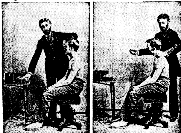
Figure 4-7. The electric-hand technique for applying faradic current in which the therapist is in series with the induction coil and patient (From Beard and Rockwell Medical & Surgical Uses of Electricity. New York 1891, W. Wood Co. 788pp.).
